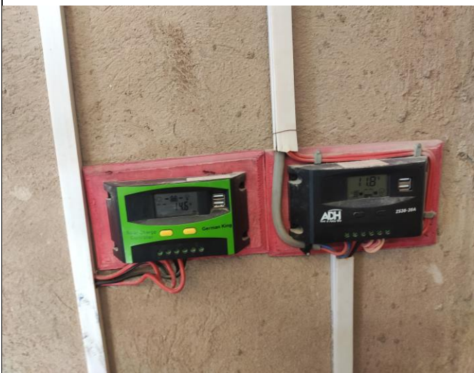
Monitoring system of growing room
