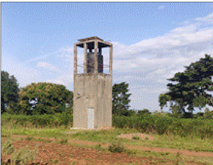
Innovation Africa Water Tower
