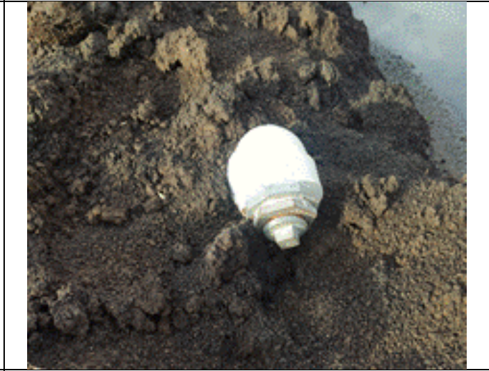
Connection of pipes for site
